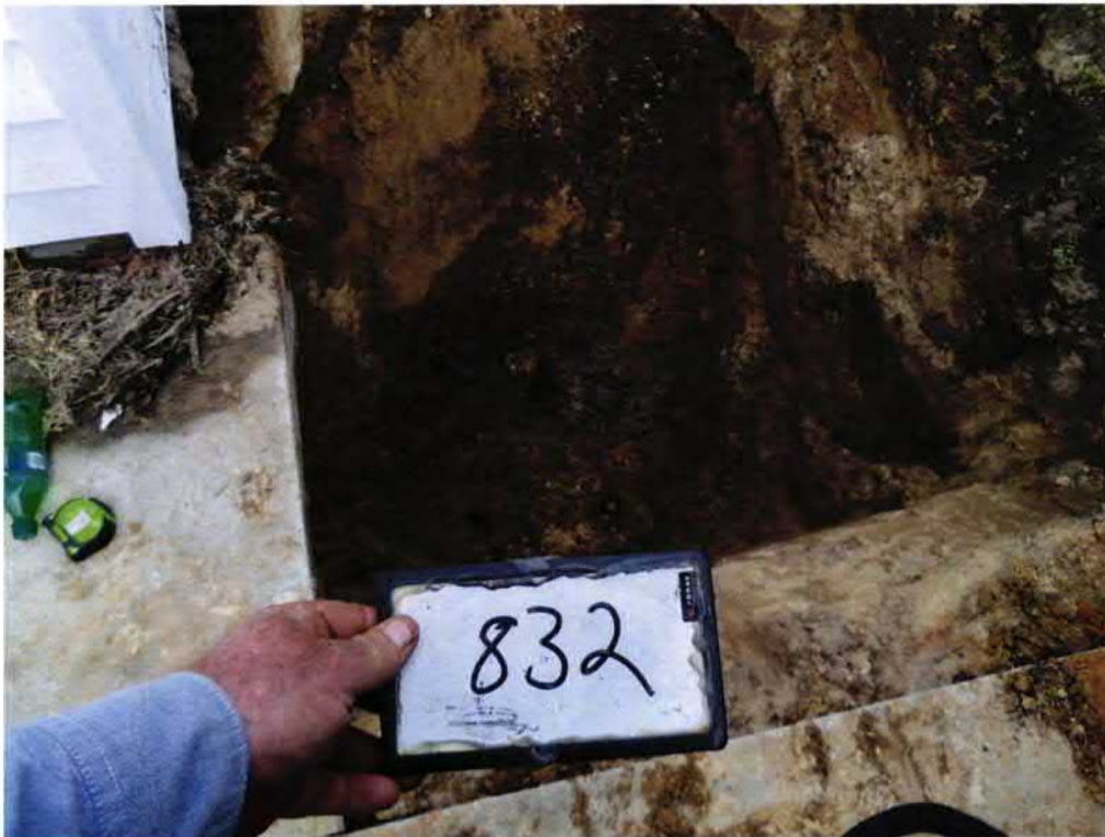
Picture 2: UST 832Azalea excavation.
